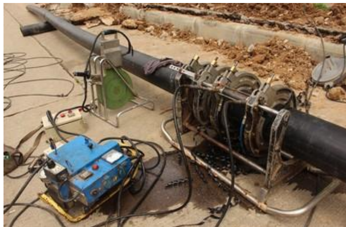
Figure 4-6 Heating of surface with heater for welding of HDPE pipe
