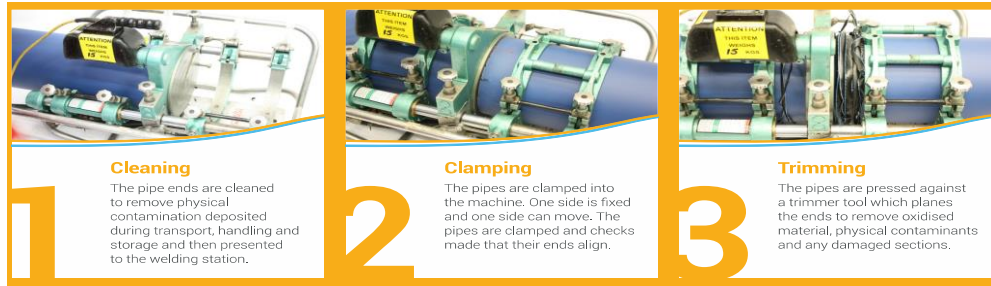
Figure 4-5 Cleaning, clamping and trimming the HDPE pipe for welding
