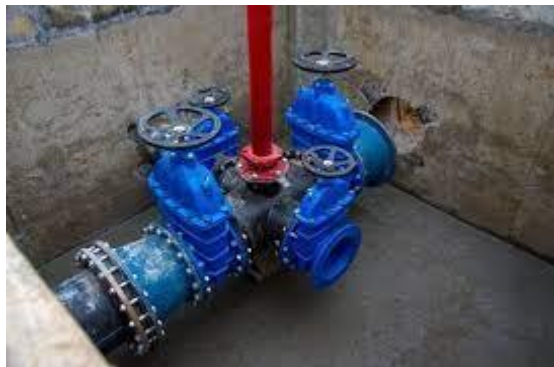
Figure 3-2 Gate Valve
