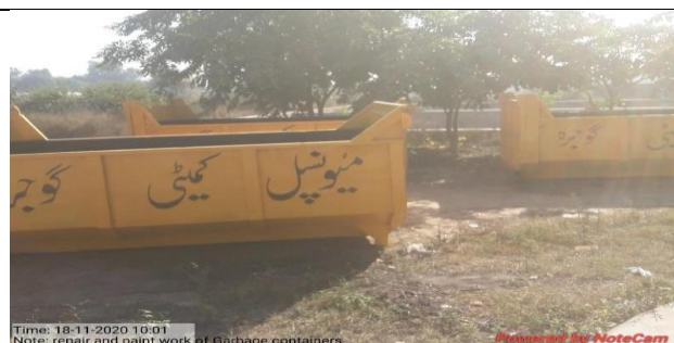
After: Garbage Containers repair
