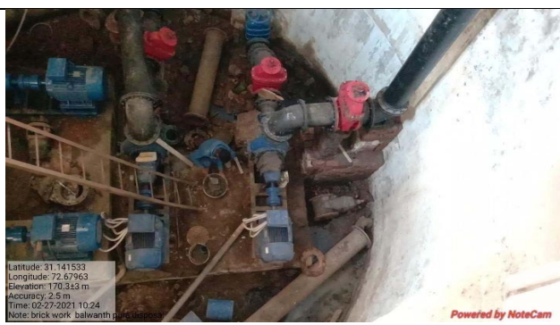
Balwant Pura Disposal Pump House after installation of Sullage Pumping Units (5 Cusec)
